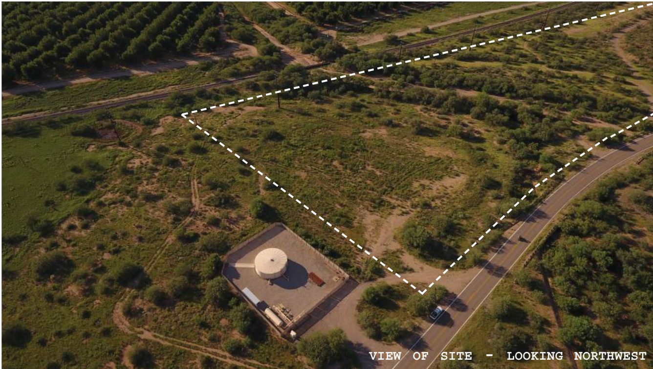
AERIAL VIEW OF SITE
